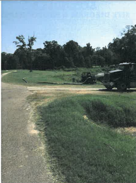
Pumping operations on Thursday July 19, 2018
