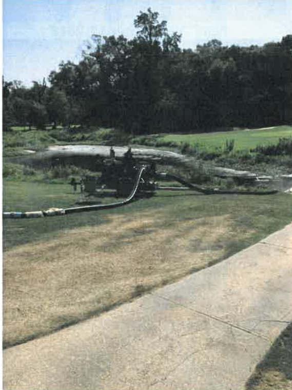
Pumping operations on Thursday July 19, 2018
