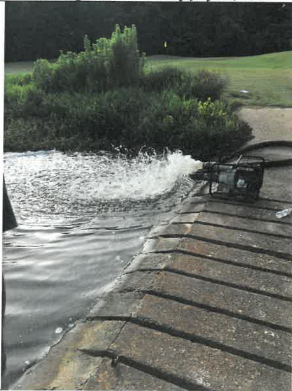
Aerating water Thursday July 19, 2018
